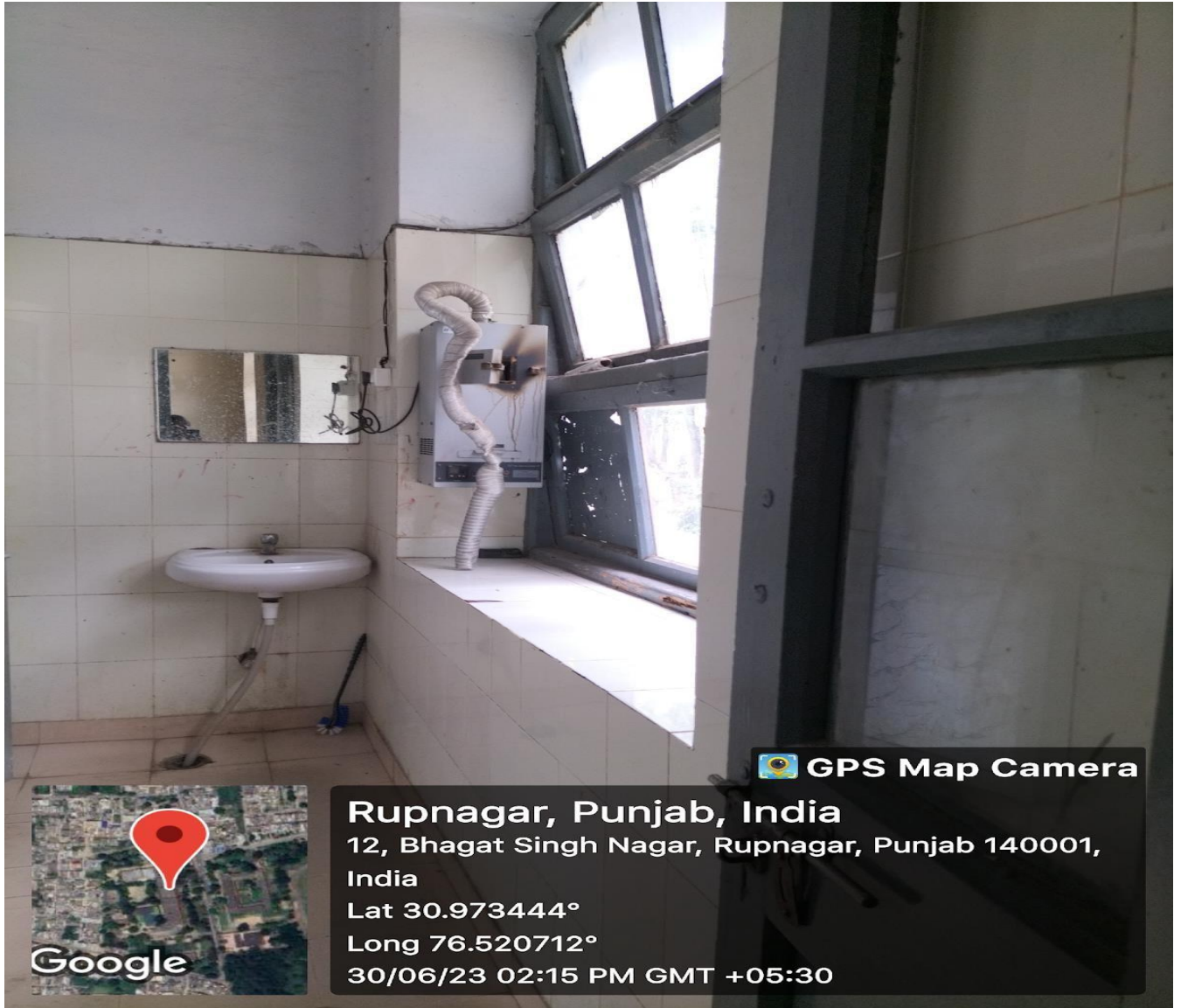
Incinerator for girls common room
